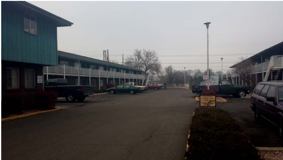
Photo No. 11: Jody Apartments to west of Property, facing south
