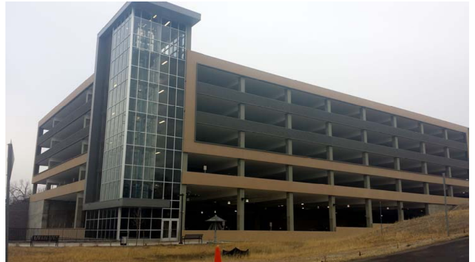
Photo No. 8: RTD parking garage, facing southwest
