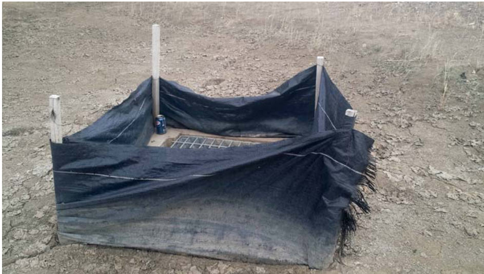
Photo No. 7: Stormwater detention drain on 1050 Ames Street parcel
