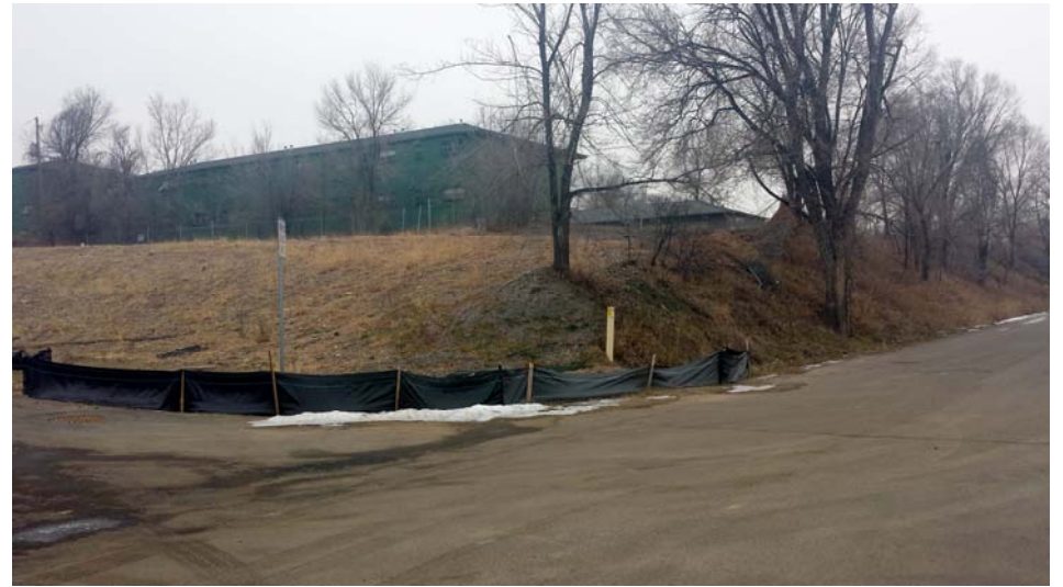
Photo No. 10: 1079 Ames Street parcel and Jody Apartments, facing southwest
