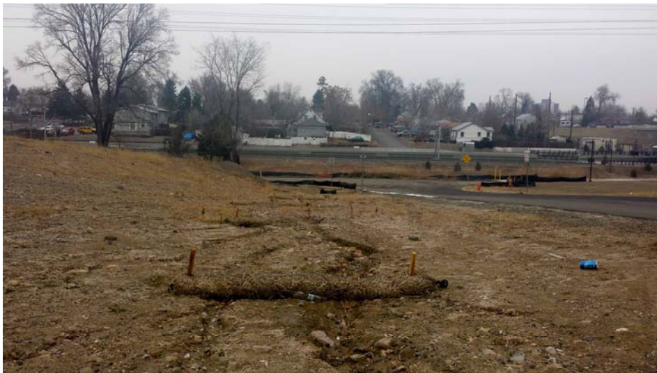
Photo No. 3: 1079 Ames Street parcel with erosion control berms, facing north
