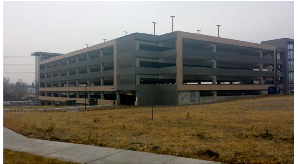
Photo No. 2: 930 RTD parking garage, facing northeast
