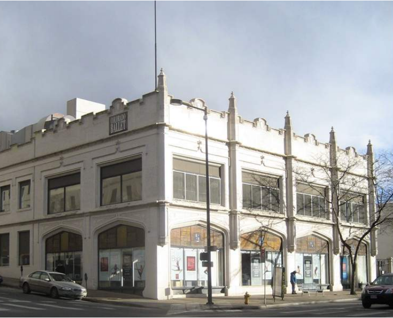
Former Colorado Ballet building owned by the State Land Board via Denver Stuff Blog
